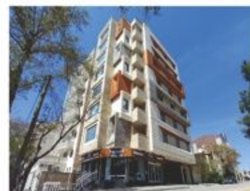
CITY STAR Building
