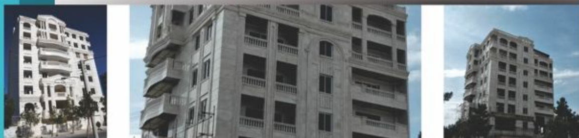
PARADISE PALACE Building
